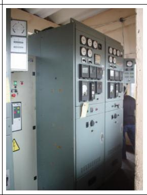
Control panel for generator 4 (although it indicates generator No. 2 at the top) and No. 3 again
